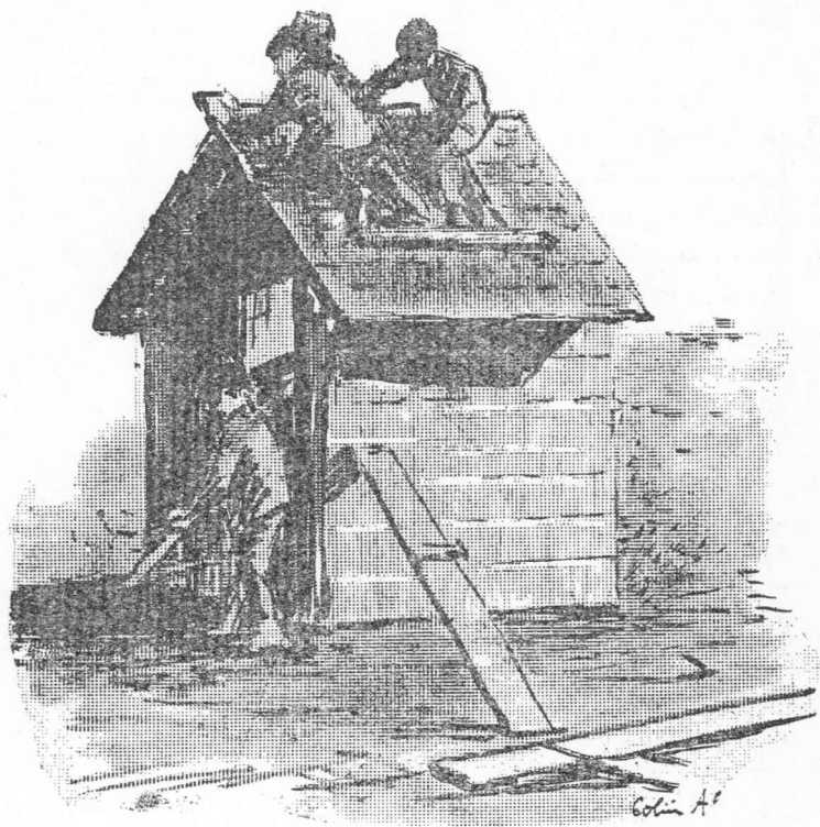
HOUSE APPROACHING COMPLETION.
