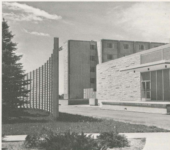
West Campus' McCowen Hall is one of the two "H" design buildings used for coeducational living. The building is a five-story structure which houses 1,044 men and women.
