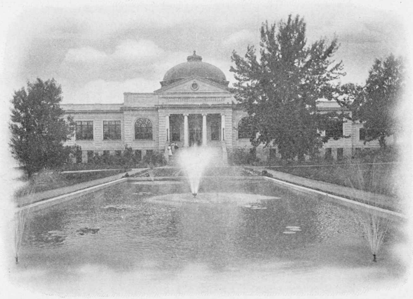
THE LIBRARY, POOL, AND FOUNTAIN.
