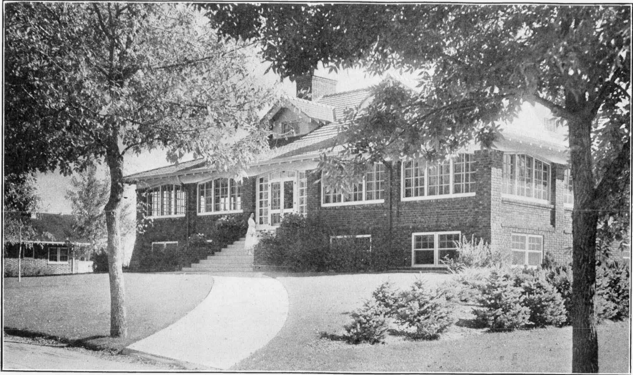
WOMEN'S CLUB BUILDING Attractive Within and Without
