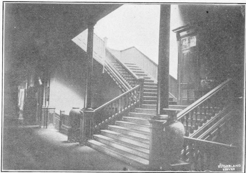
Stairway to Third Floor.
